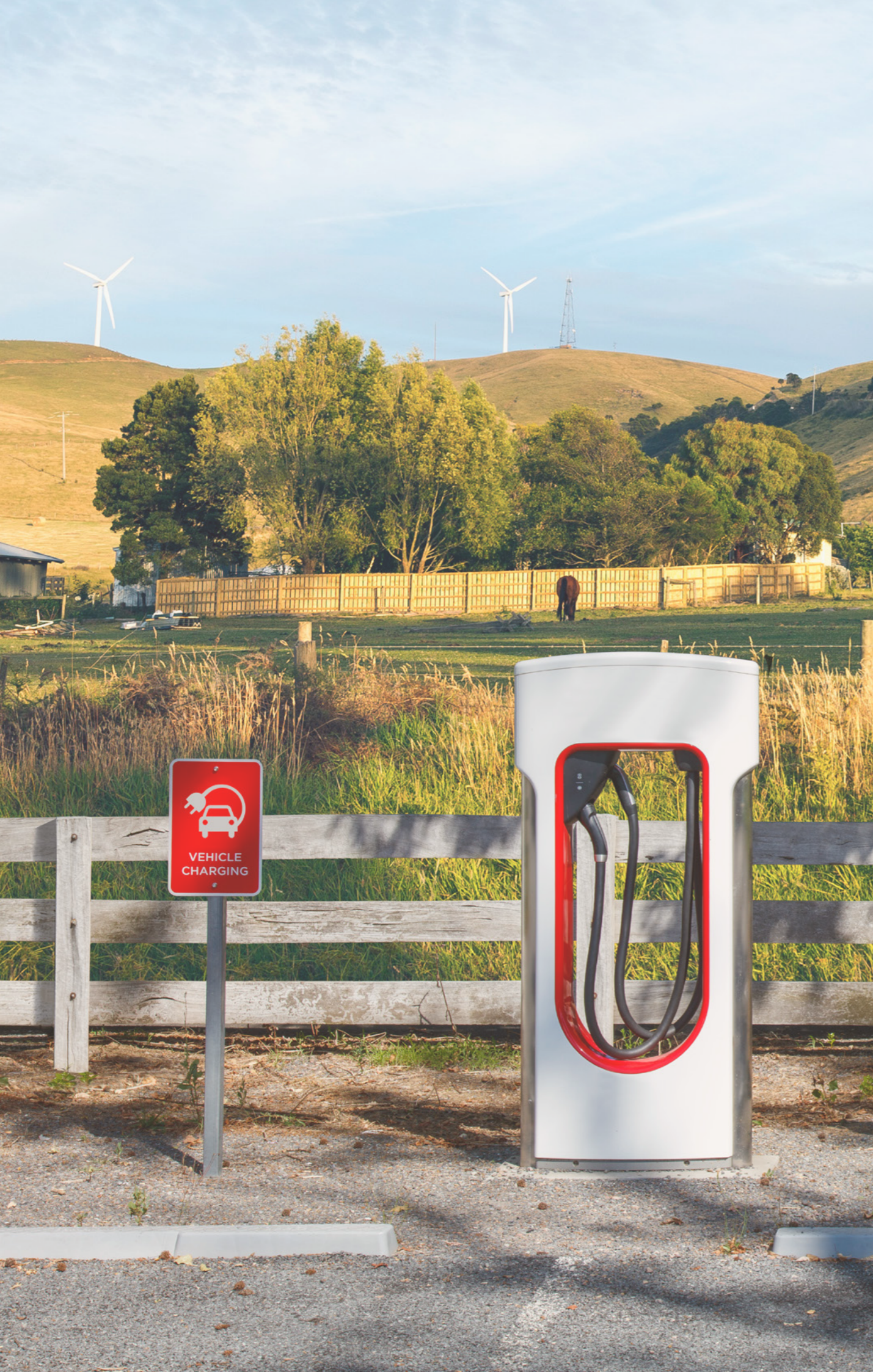
▲ Remote electric vehicle charging station, VIC
