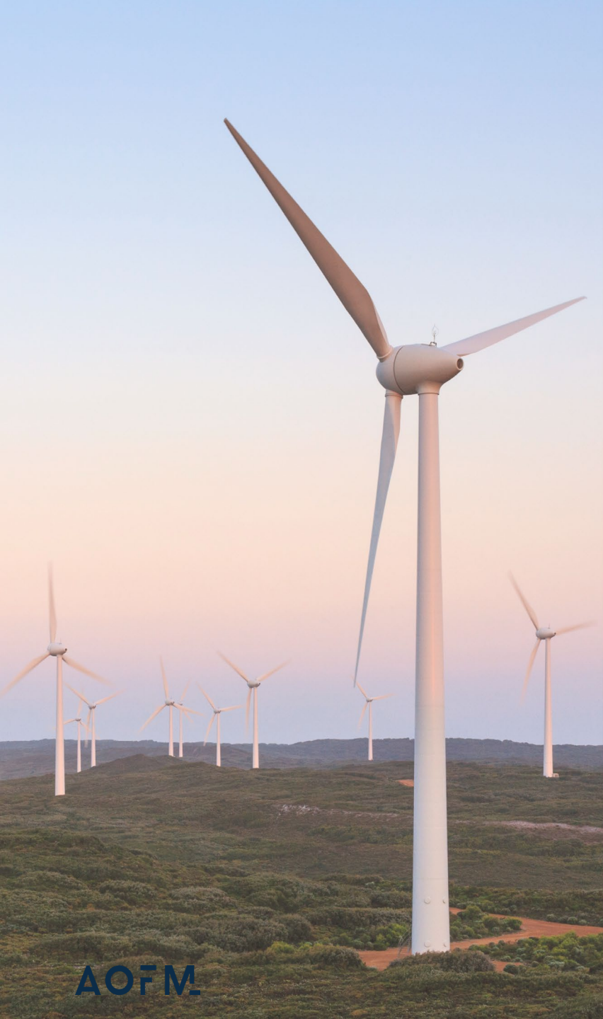
▲ Albany Wind Farm, Albany, WA
